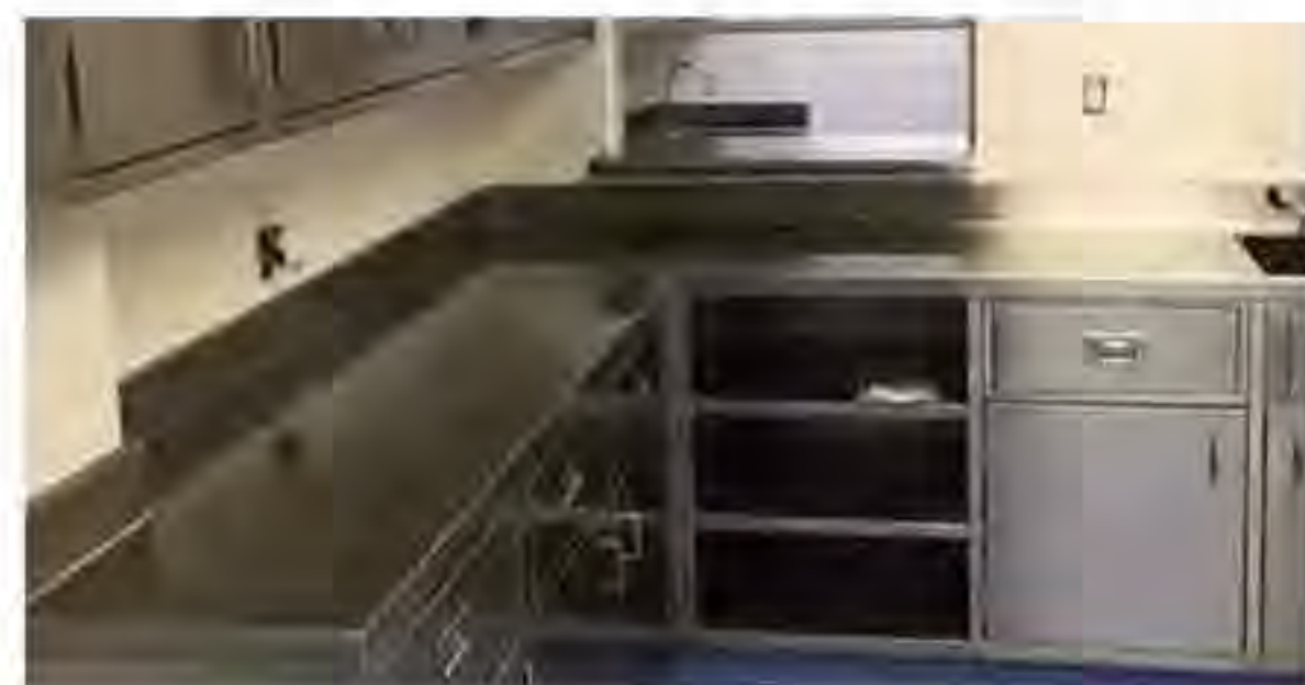
stainless steel countertops fabricated to drawings indicating backsplash height, raised edge and field condition requirements
